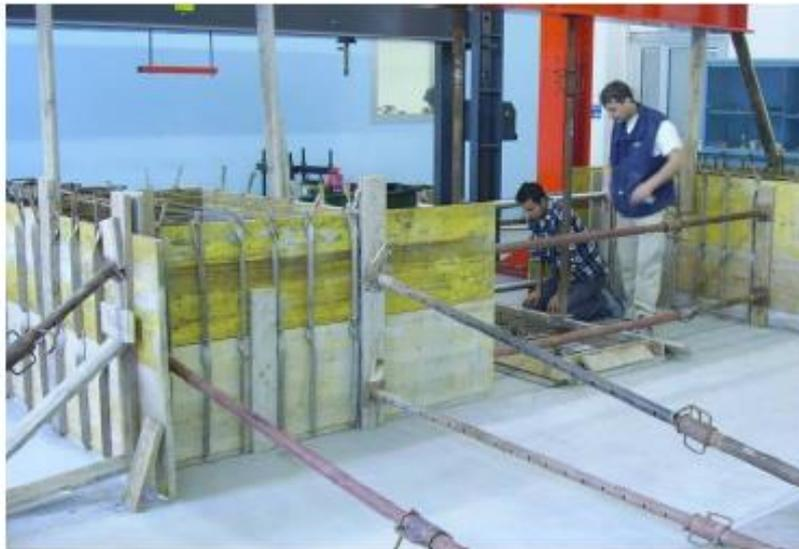
Figure 92. The arch bridge model construction: reinforced concrete blocks formworks
