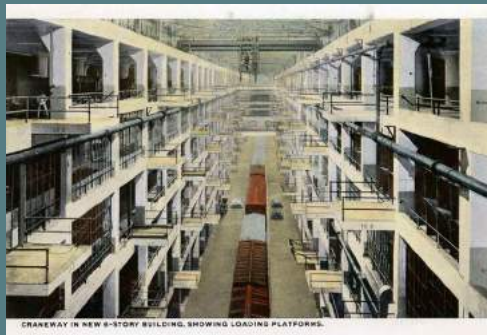
CRANEWAY IN NEW 8-STORY BUILDING, SHOWING LOADING PLATFORMS.
