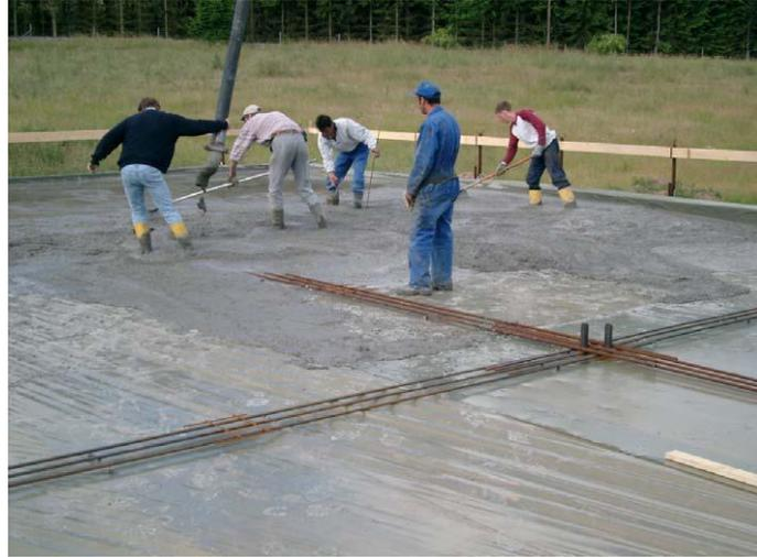
Figure 16: Construction of the full-scale HRFA slab test in Bissen, 2004 [9]
