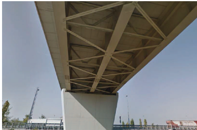
Figure 3.7: Bracing systems view Source: https://www.google.it/maps
