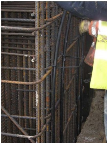
Figure 3.11 Coupling of the pipes to the cage (Amis et al.,2010)
