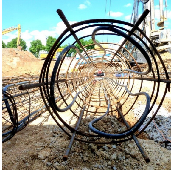
Figure 3.2 Energy Pile (Brandl, 2006)
