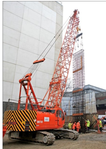
Figure 3.10 Inserting the geothermal pipes into the diaphragm cage (Amis et al., 2010)
