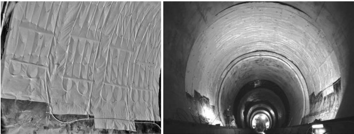
*Figure 1.9. Energy geotextile installed in an energy tunnel - conventional tunnelling method – Lainzer Tunnel Vienna (Adam & Markiewicz, 2009)*
