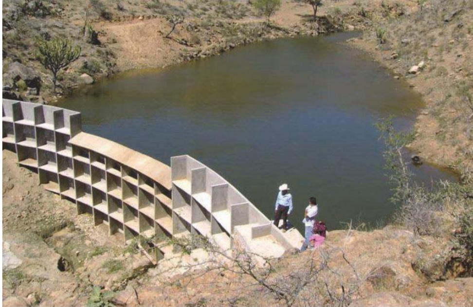
**Figure5. 13:** Ferro-cement Storage Reservoir
