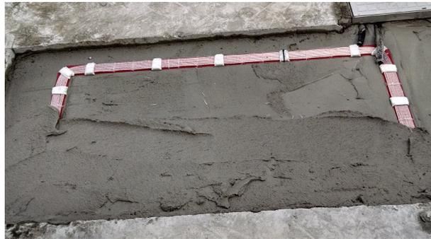
Figure 2.1: Coil embedding with a layer of 2 cm of concrete [3].
