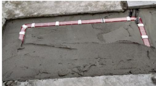
Figure 6.1: Road embeddment of the 9 turns WPT in dry concrete.
