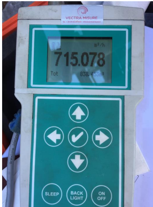
Figure 3.3: Portable flow meter display after the water to thickener flow measure.
