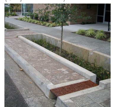
WADI a Portland, Stati Uniti (Greywater Action)
