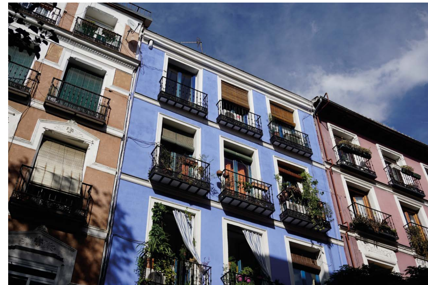
Plaza Augustin Lara - 2018 // Typical buildings in Lavapiés - 2018
