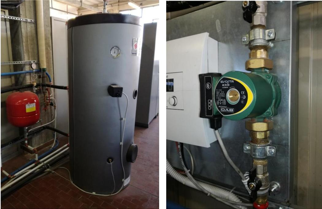
**Figure 28 – Water tank and water pump of the secondary loop**
