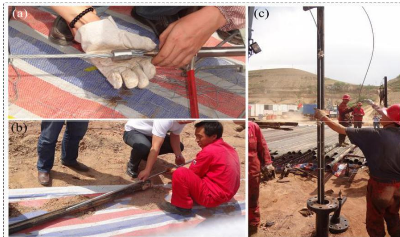
Figure 12. Well-logging field: (a) Downhole cable; (b) Tied to the downhole tube; (c) Sensor down well process.
