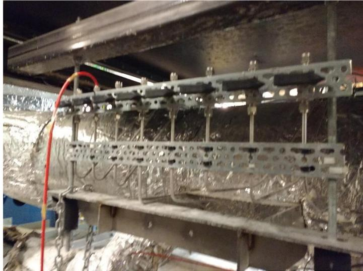
Figure 21 Picture of the valves for the purge system.
