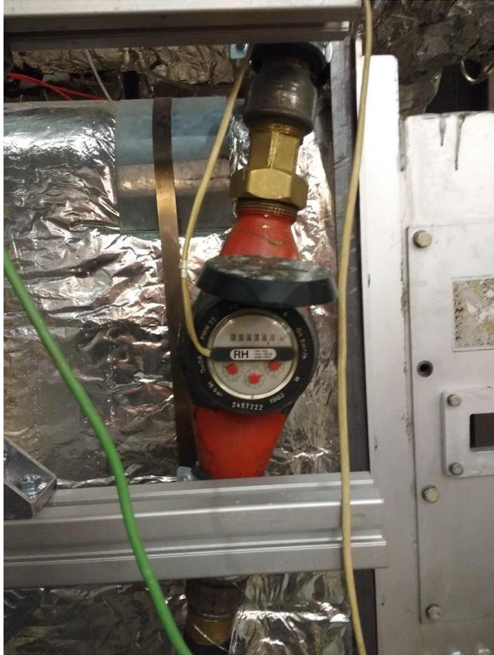
*Figure 27 Picture of the volumetric flow rate counter..*
