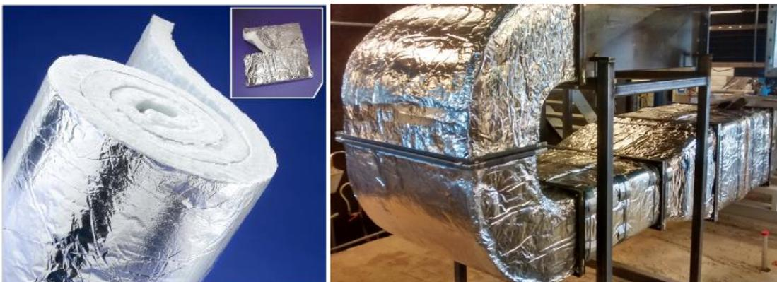
Figure 22 Insulation material and picture of the insulated ducts. [1]
