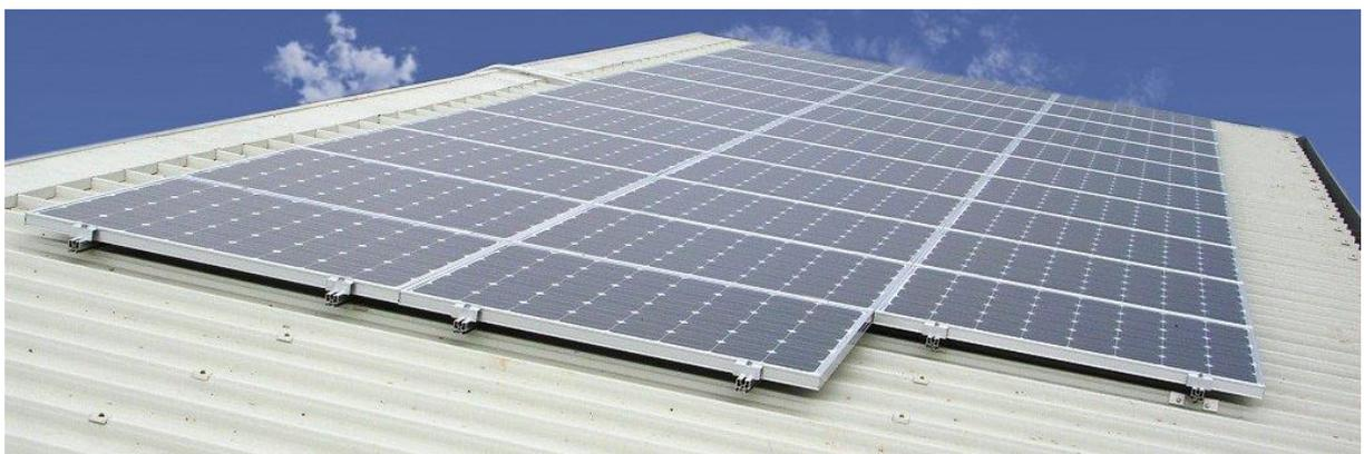
Fig 5.6: Example of PV panels on corrugated sheets ([www.puntoenergiashop.it](http://www.puntoenergiashop.it)).
