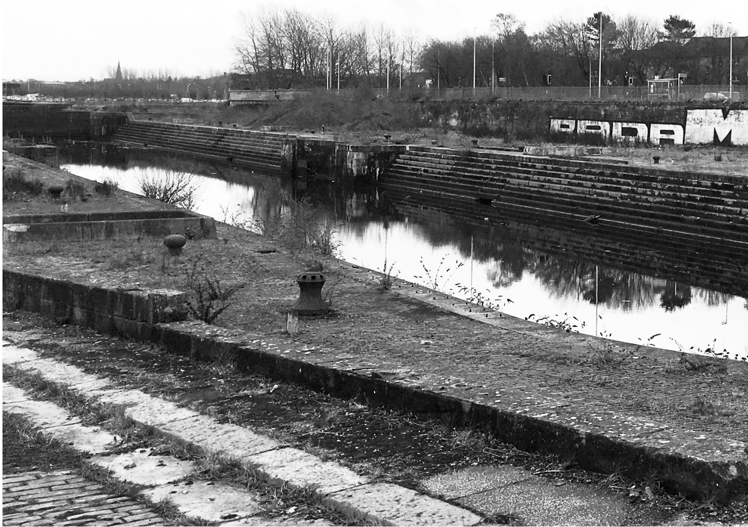
Figure 4.6 | Dock 3. Govan Graving Docks.
