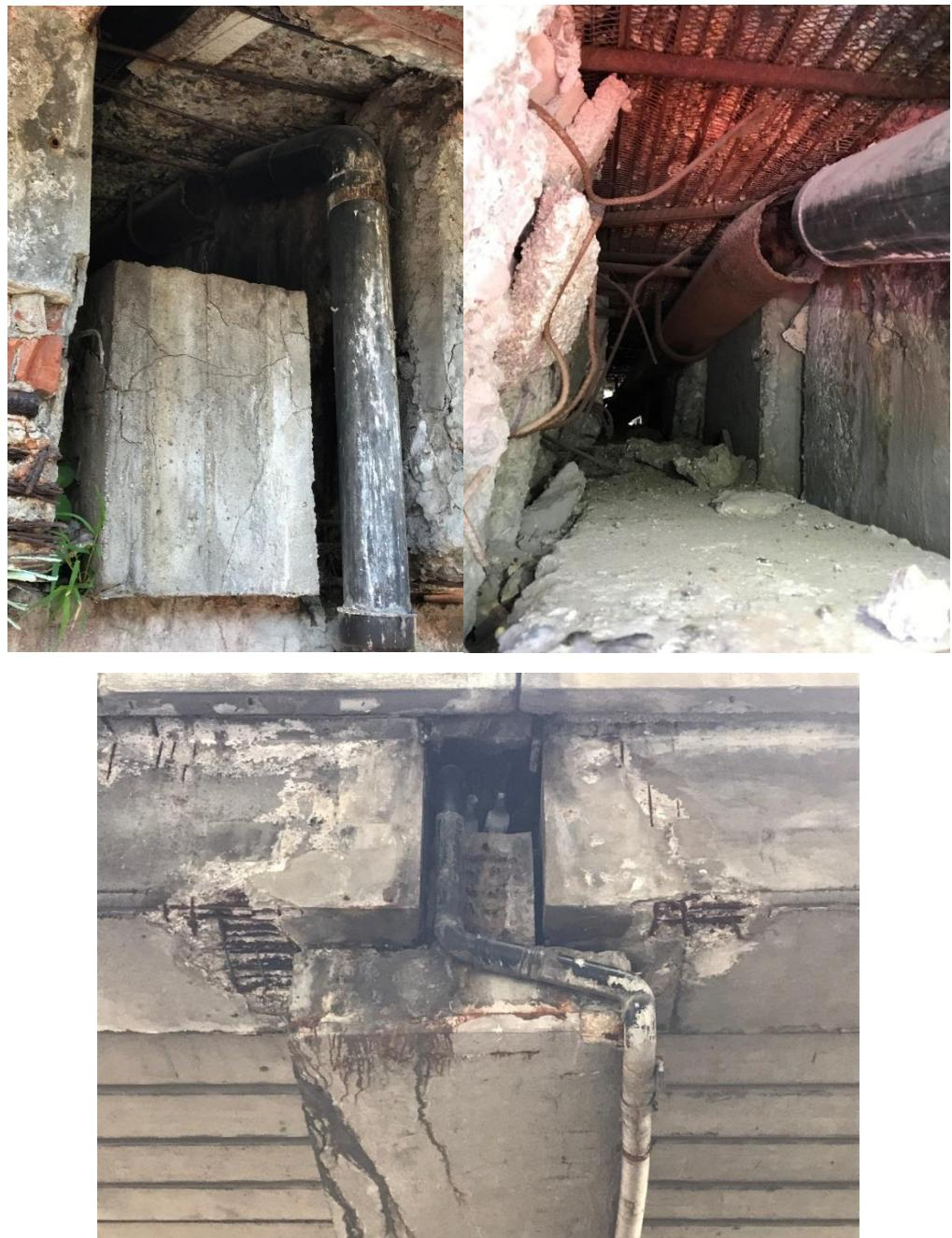
*Figure 53 Examples of the problems at the drainage channels detected.*
