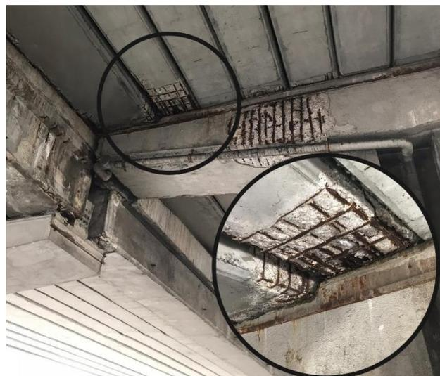
*Figure 49 Examples of the corroded outermost I beam*
