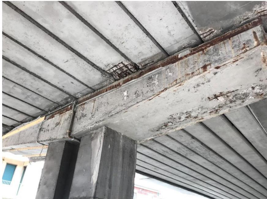
*Figure 52 Corrosion of an intermediate beam*
