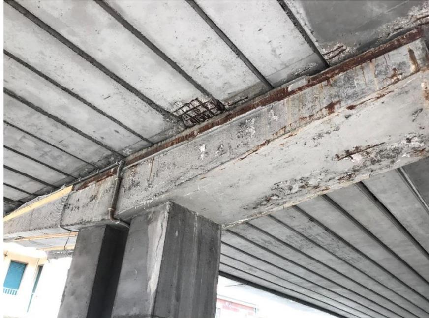
*Figure 52 Corrosion of an intermediate beam*
