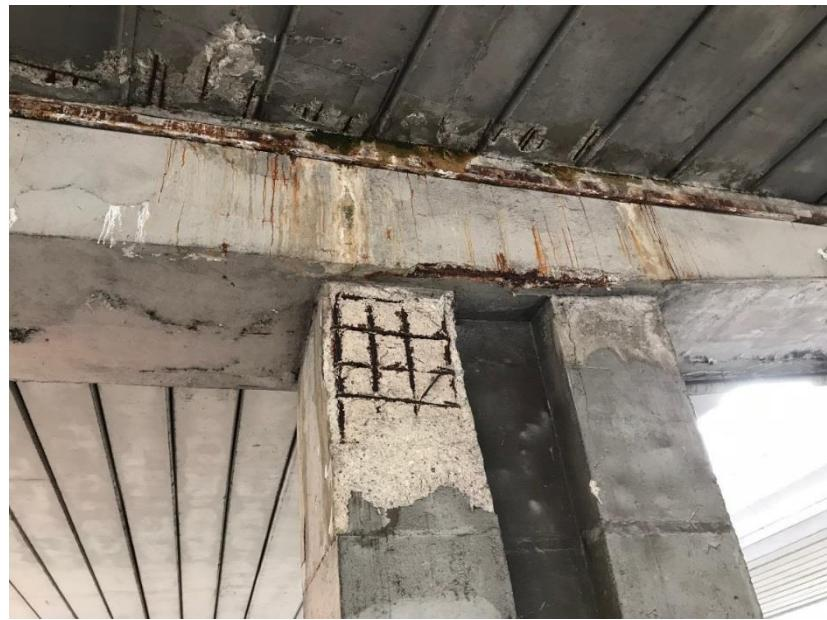
*Figure 54 Clear corroded beams close to the support*
