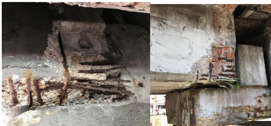
*Figure 55 Supposed support loss because of strong corrosion state*
