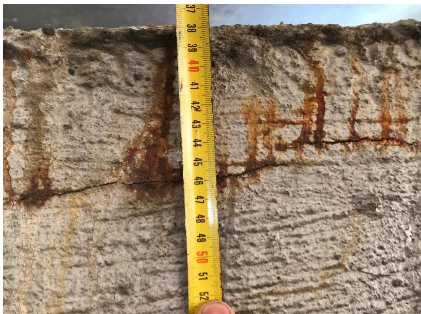
*Figure 51 Distance of a longitudinal crack from the edge*
