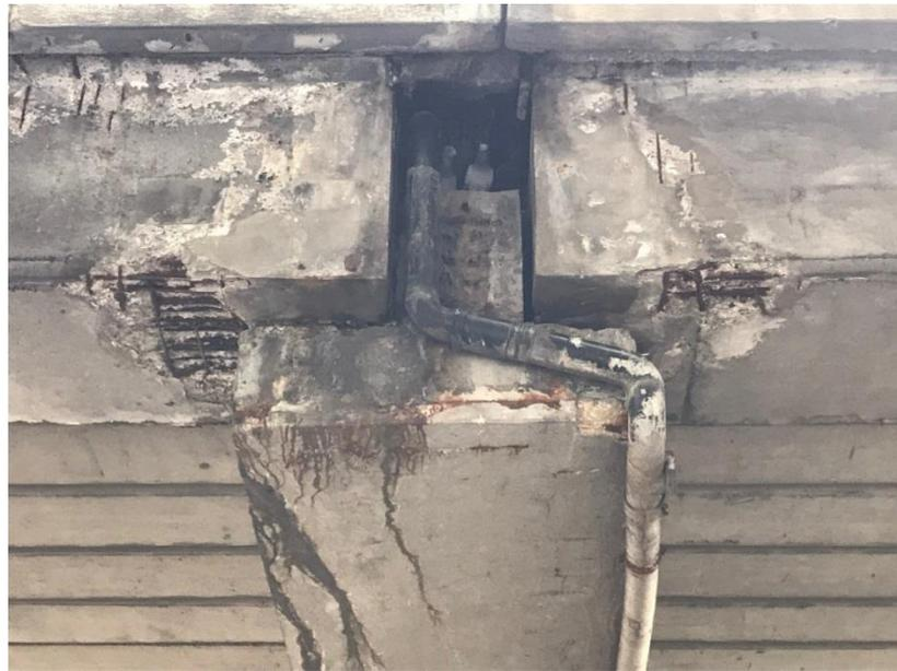
*Figure 53 Examples of the problems at the drainage channels detected.*
