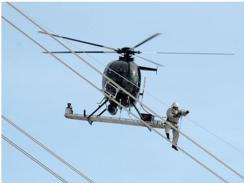
Figure 6 – Power line inspection of cable and main structure maintenance.
