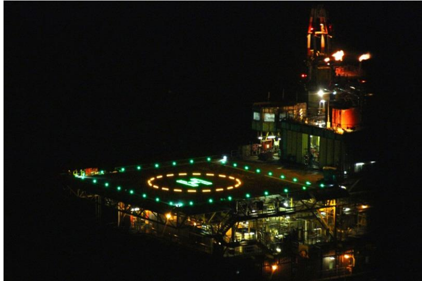
Figure 30 – Helideck Lighting System.
