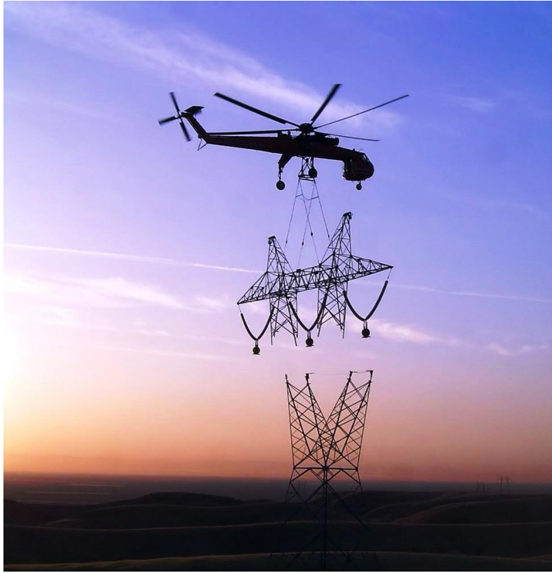
Figure 4 – S-64 Skycrane during posing operation of a powerline.
