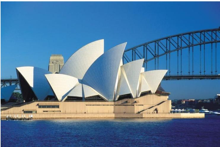
**Figure 1.3:** The Sydney Opera House (designed by Jørn Utzon and inaugurated in 1973) comprises three groups of interlocking vaulted shells which are set upon a vast platform and are surrounded by terrace areas that function as pedestrian concourses
