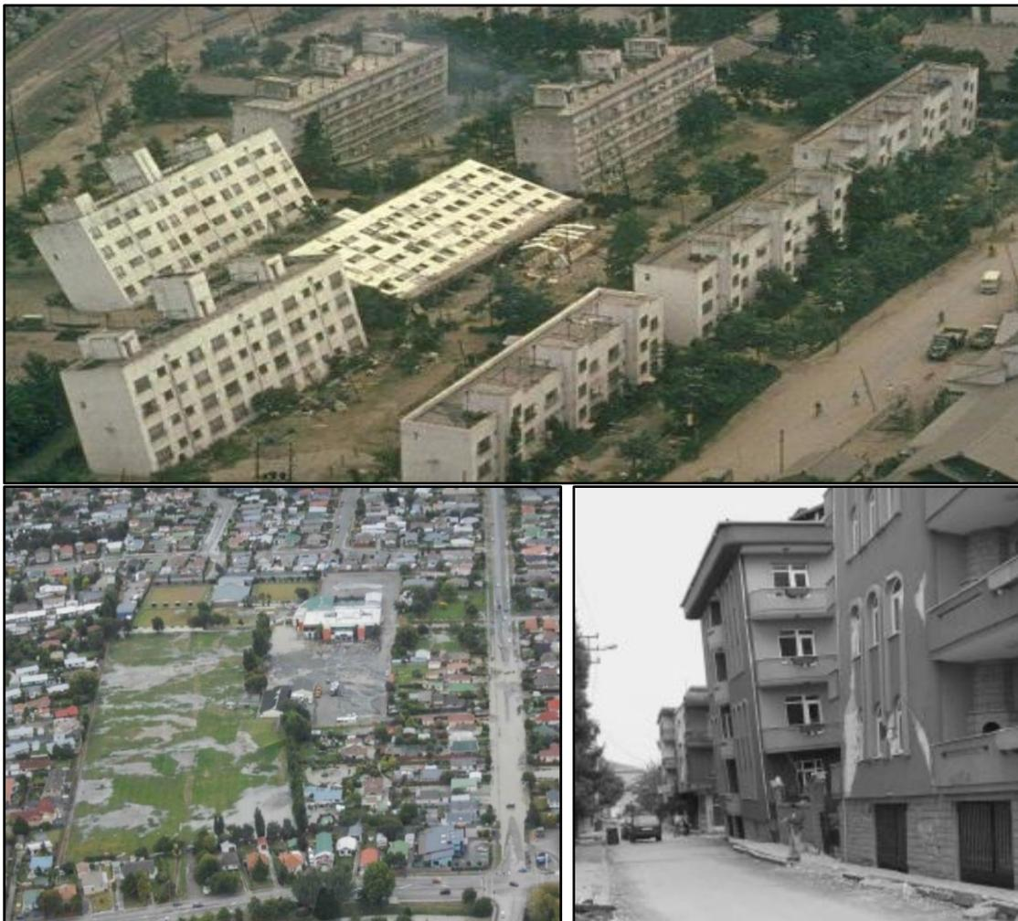
Figure 2.1- (a) Liquefaction induced rigid tilting after 1964 Niigata earthquake; (b) Liquefaction in a residential area of Christchurch, from Diaz, 2016; (c) 5-storey building tilting after Adapazari earthquake, Turkey, from Bray et al., 2001.
