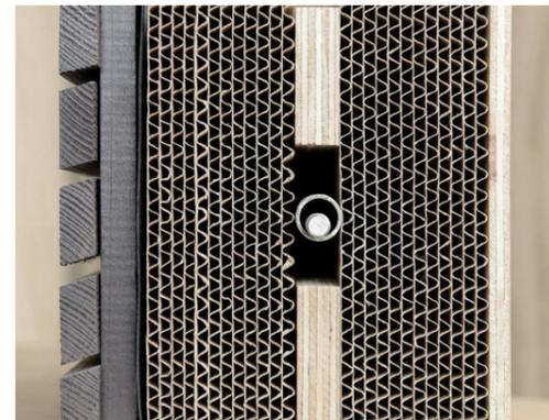
FIGURA 5.49: SCHEMA DI ASSEMBLAGGIO DEI MODULI DELLA WIKKLE HOUSE
