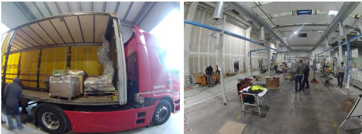
The equipment arrived at the plant via 3 trucks loaded with all the material in the last two days of production before the holidays and was offloaded and stored in stockage bays. The installation then started with the removal of the shutter conveyor along the final lines. Laser measure instruments were employed to trace the layout of all the automation stations on the floor, then holes were drilled in the ground in correspondence of the fastening points for
