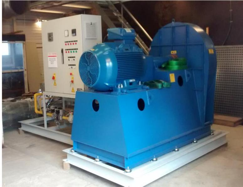
*Figure 32. Hot air generation unit placed in the room where the test bench has been built.*
