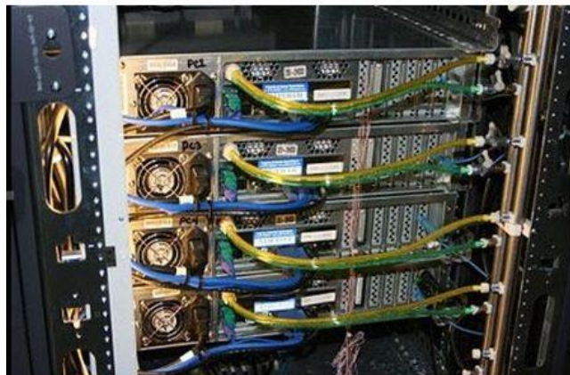
Figure 15- Direct to the chip cooling system ( http://www.tomsitpro.com )
