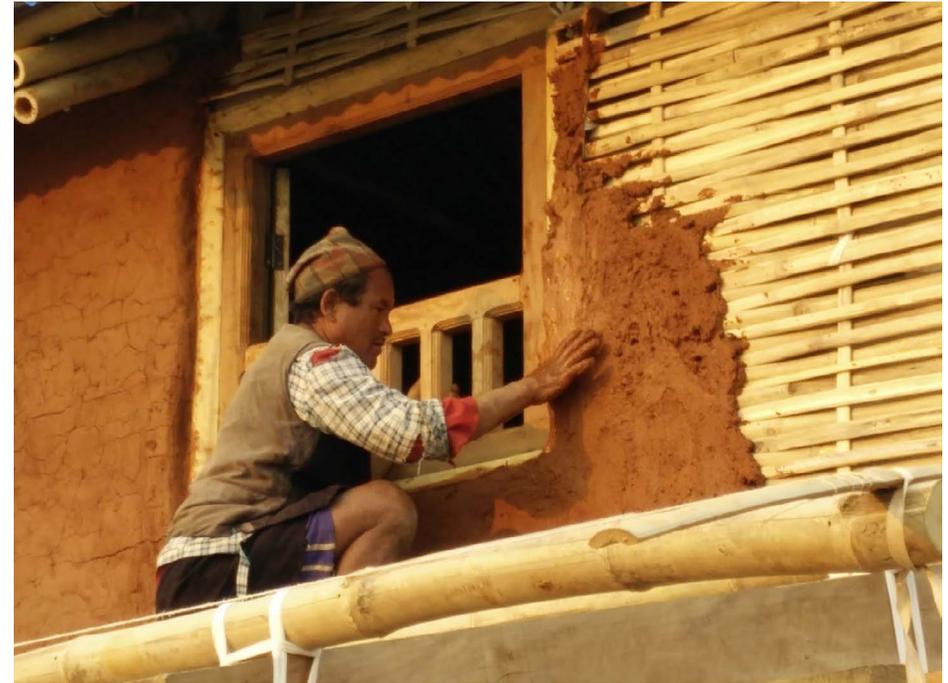
Fig 5.19 Posa rivestimento in terra-paglia wattle-daub (thekauleprototype)
