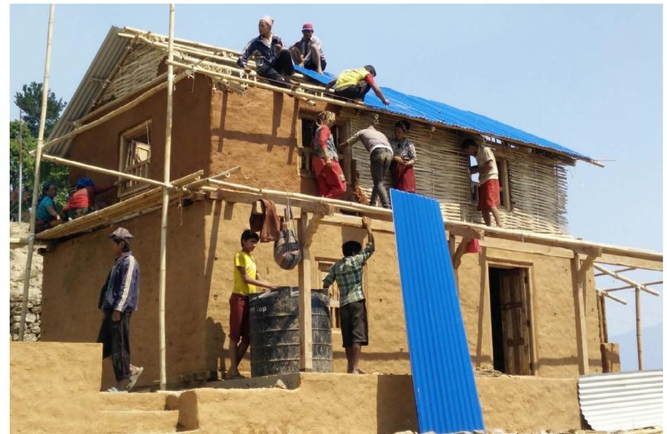
Fig 5.20 Posa rivestimento in terra-paglia wattle-daub (thekauleprototype)
