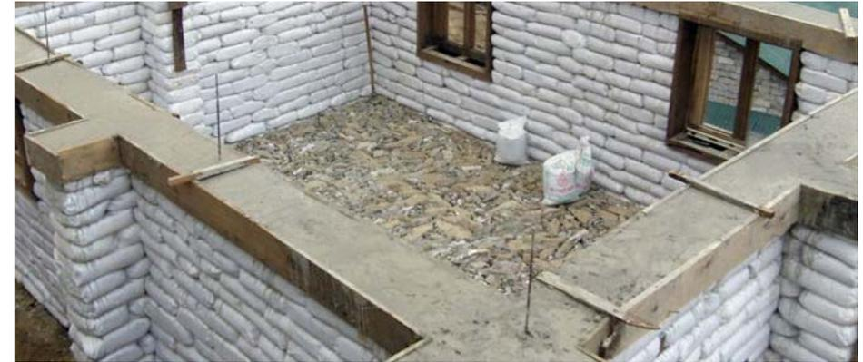
Fig 4.41 Cordolo superiore in cemento armato (DG vol ii)
