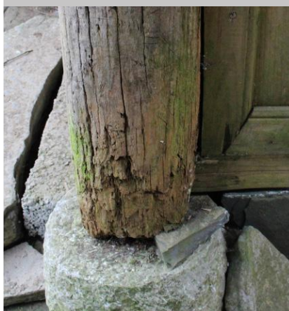
Fig.4 Detail of a stone foundation-pillar joint.
