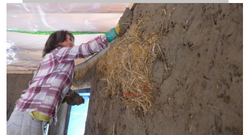
Fig.9 Straw bale wall being plastered with lime render.
