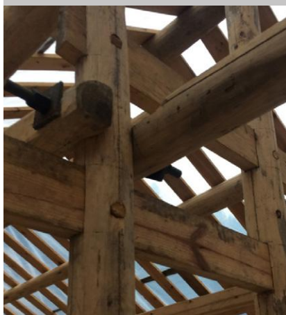
Fig.3 Contemporary reproduction of the traditional mortise and tenon joints typical of the traditional Miao house.
