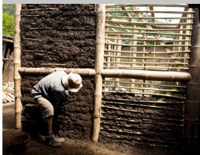
Fig.5 Bamboo skeleton of a bajareque wall.
