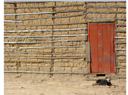
Fig.2 A bajareque wall cracked because of shrinkage.
