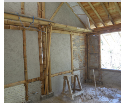
Fig.3 Bajareque wall with lime infill.
