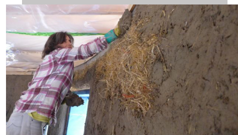
Fig.9 Straw bale wall being plastered with lime render.
