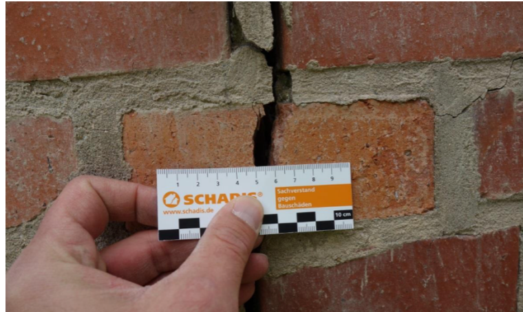
Fig. 7.3: Crack width of the vertical crack
