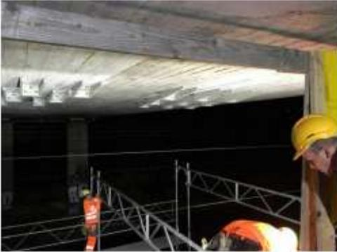
Figure 01: Mobile scaffolding structure
