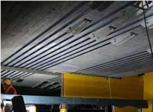
Figure 02: Tensioned StressHead CarboStress<sup>®</sup> systems
