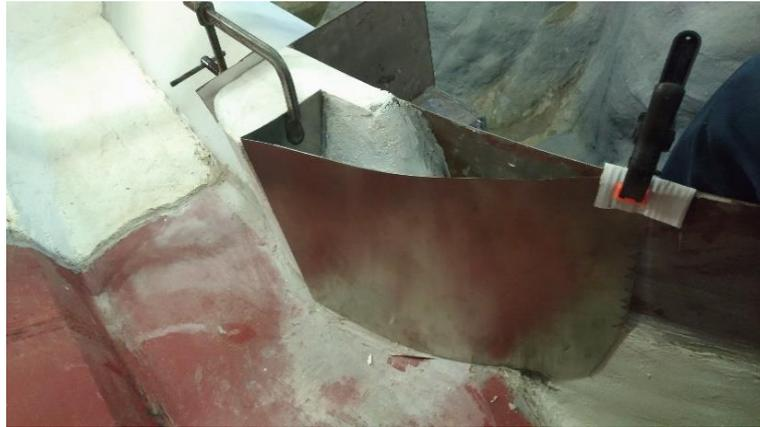
*Figura 24 raccordo curvilineo in inox*
