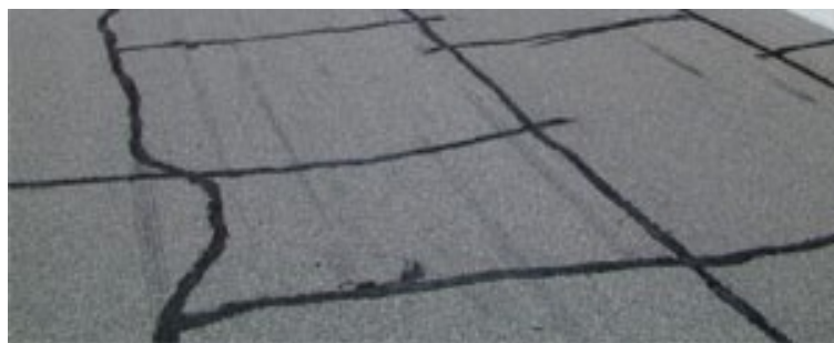
Figura1.2 block cracking
