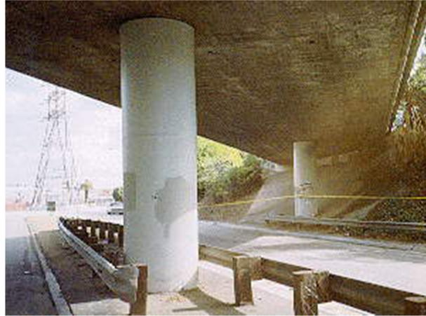
*Figure 2.12 – Steel jacketing of pier:
