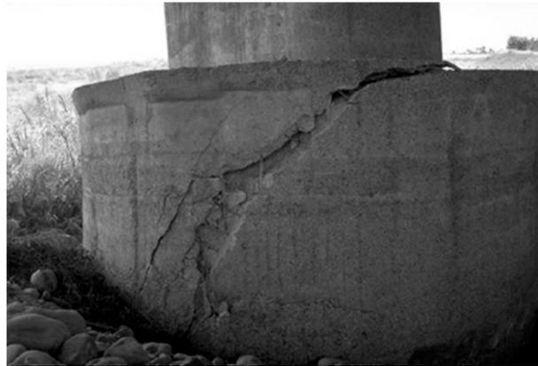
Figure 2.20 – Foundation collapse: Chi Chi earthquake, Taiwan, 1999
