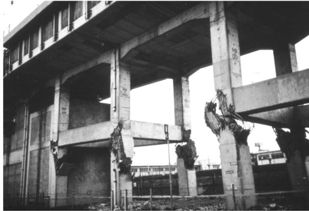
Figure 2.10 – Kobe earthquake, Japan, 1995, Shinkansen Viaduct (Pinto, Franchin, & Lupoi, 2009)
