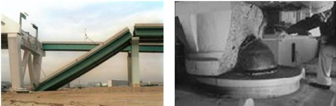
*Figure 2.2 – Kobe earthquake, Japan, 1995: a) Unseating, Nishinomiya-ko Bridge and b) Bearing failure, Higashi-Kobe Bridge (Pinto, Franchin, & Lupoi, 2009)*
