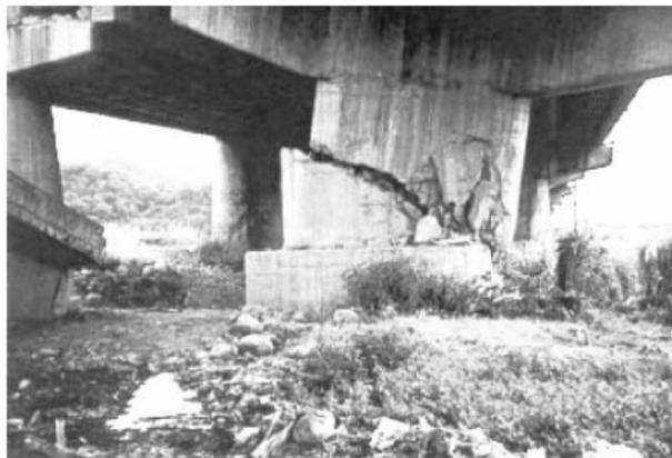
Figure 2.8 – Chi Chi earthquake, Taiwan, 1999, Wushi Viaduct: column shear failure (Pinto, Franchin, & Lupoi, 2009)
