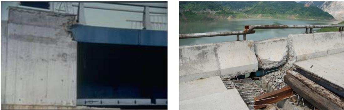
*Figure 2.4 – Pounding damage:
