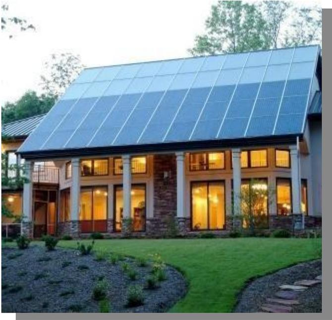
*This North Carolina home gets most of its space heating from the passive solar design, but the solar thermal system supplies both domestic hot water and a secondary radiant floor heating system.*
