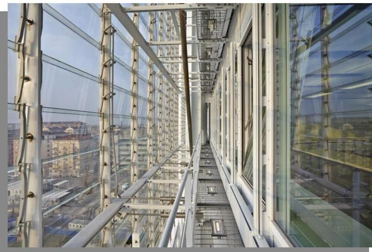
Figure 2.18 – ventilated and automated facades
