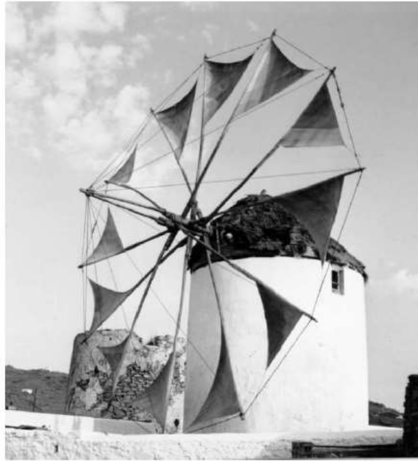
Figure 3: Greek tower mill, with "yawing". Source: Hau, wind turbines fund, p.8.
