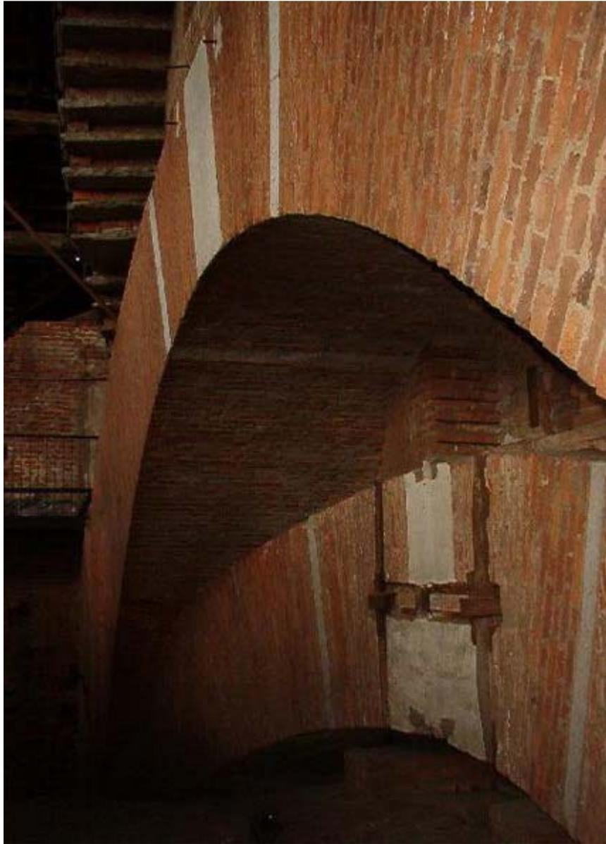
The impost arches of the dome of Novara, a complex, daring and brilliant solution to transfer loads to the below pylons (Sabrina Fassi)
