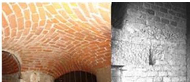
Two examples of the most important architectonic and constructive techniques: the “funnel vault” or “fungus vault”, perfectly adaptable to the “Antonelli’s system”, and stone put into the brick wall (Sabrina Fassi)
