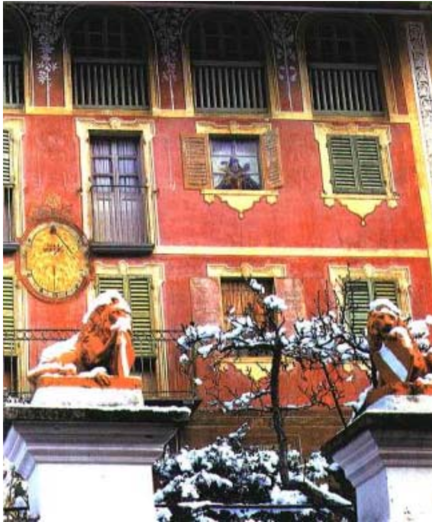
Front detail of Bottino mansion in Bonzo (Groscavallo)
