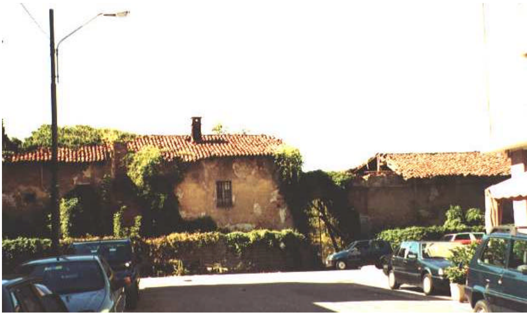
Fig.3 The Cascina Grangia farm in its present state of decay
