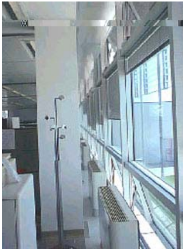
Details of the building's openings ("I Guzzini di Recanati")
