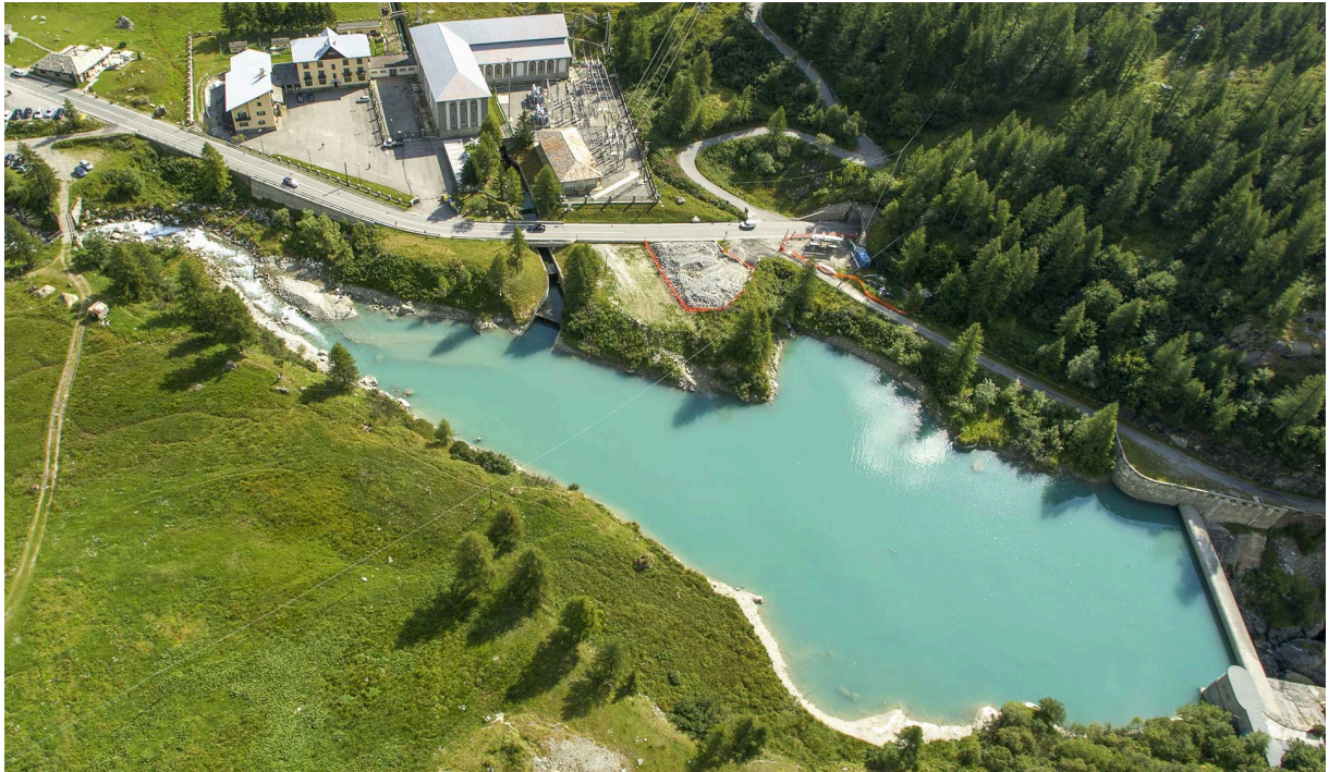
Figure 3.1 — Aerial view of the Perrères Dam reservoir, Valtournenche (AO), Valle d'Aosta. The turquoise reservoir, concrete gravity dam wall (bottom right, height 24.36 m), and hydroelectric powerhouse (top left, 18 MW) are visible. The red-outlined area indicates dredged sediment accumulation — the precursor material collected for this study. (Source: CVA S.p.A., www.cvaspa.it , 2021. All rights reserved CVA S.p.A.)
