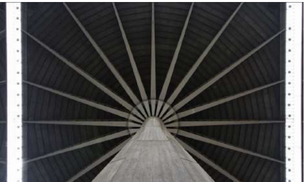
Figure 2.8: Umbrella columns defining the buildings architecture
