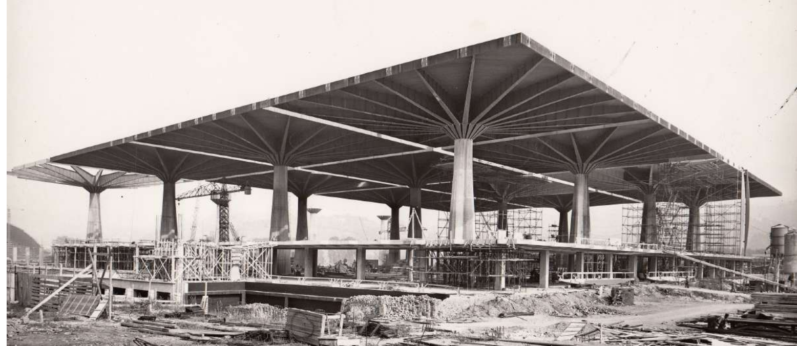
Figure 1.9: Palazzo del lavoro under construction "Courtesy of Fondazione MAIRE - ETS. Materials from the MAIRE Historical Archive."
