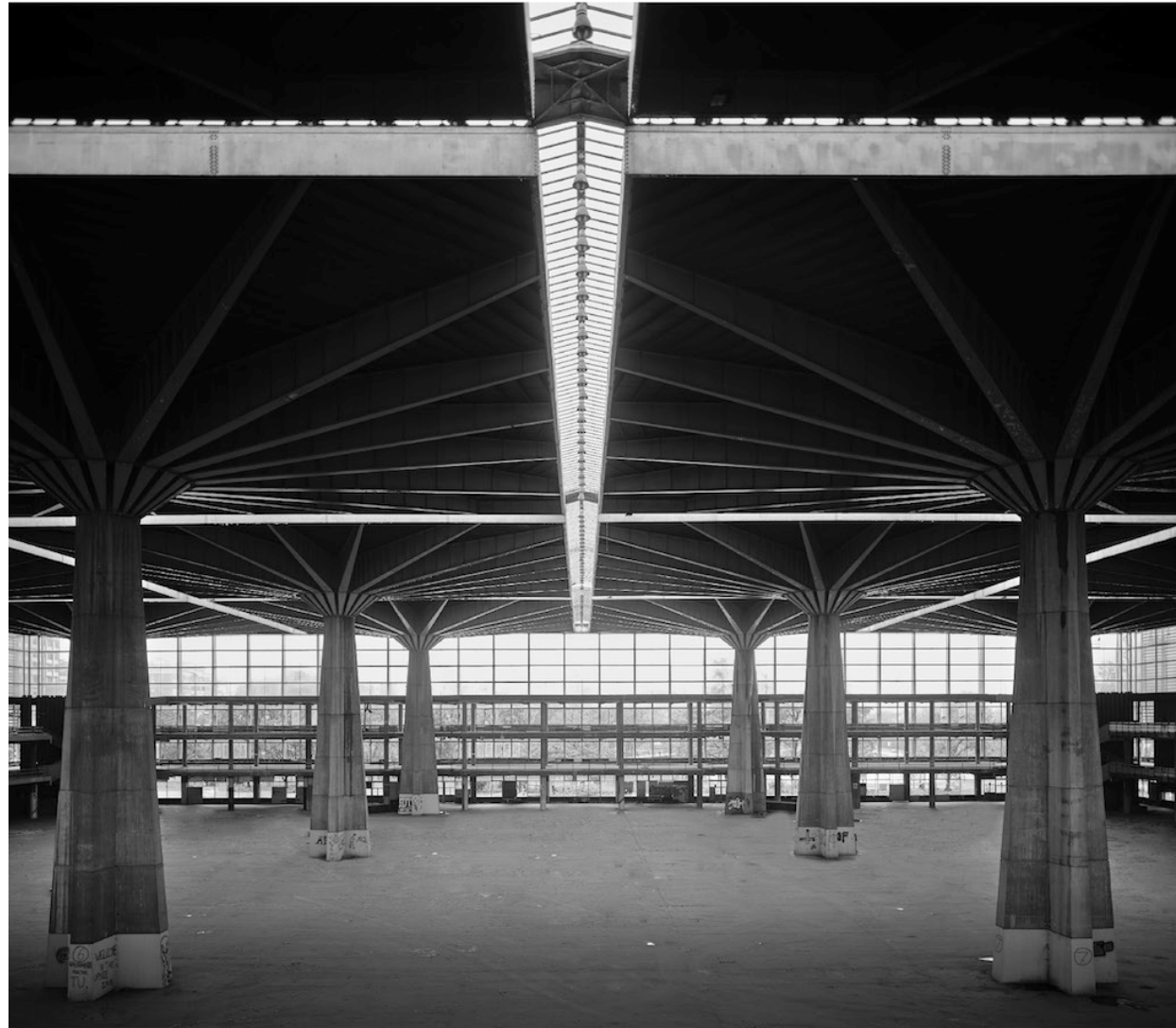
Figure 4.44: Historical archive photograph showing the raw interior volume of the main hall prior to intervention, focusing on the unaltered structural configuration of Pier Luigi Nervi's columns and roof grid.
