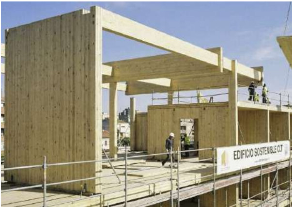
Figure 4.17: CLT Construction
