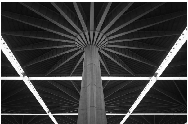
Figure 2.20: Detailed picture of an umbrella column.
