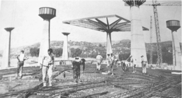
Figure 3.13: Historical construction photographs illustrating the casting process and geometry of the monumental reinforced concrete ribbed gallery slabs.
