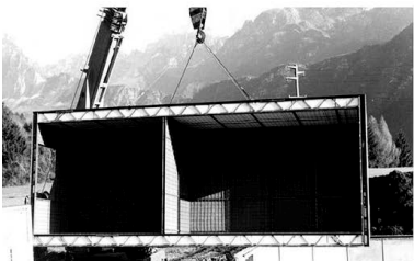
Figure 0.8: From the top, the assembly of a house with "Block-Volume" produced in the factory and plastered on site in the first years after the 1976 earthquake.
