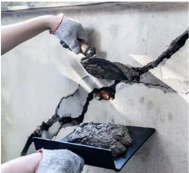
Figure 3.17: Manual application of shrinkage-compensated, thixotropic, fiber-reinforced mortar during localized micro-concrete recasting to restore structural concrete cover without altering original column geometry.
