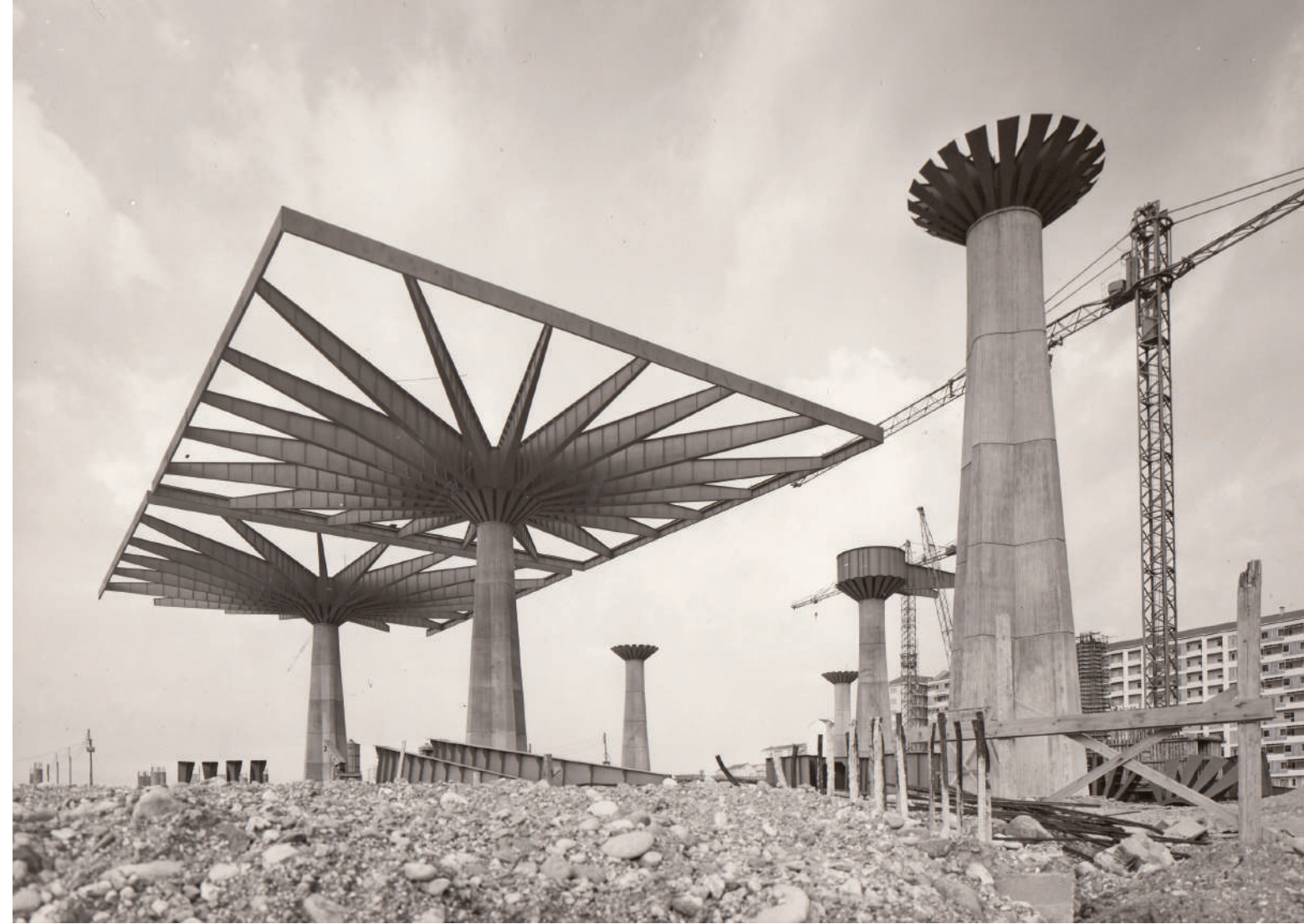
Figure 3.10: Palazzo del Lavoro roof under construction "Courtesy of Fondazione MAIRE - ETS. Materials from the MAIRE Historical Archive."
