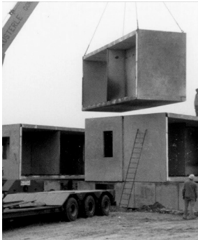
Figure 0.7: Left: "Block-Volume" laid on formwork panels forming the basement floor. Middle: production and assembly of a "Block-Volume" element forming part of the villas plastered in the factory in the post-1985 period. Right: tipping of the "Block-Volume" using an overhead crane.
