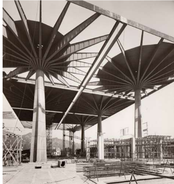
Figure 1.8: Palazzo del lavoro under construction "Courtesy of Fondazione MAIRE - ETS. Materials from the MAIRE Historical Archive."
