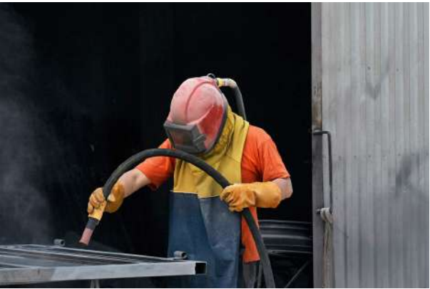
Figure 3.20: Controlled abrasive blasting using aluminum oxide media on structural steel to achieve an Sa 2½ surface preparation grade prior to the application of the high-durability coating system.
