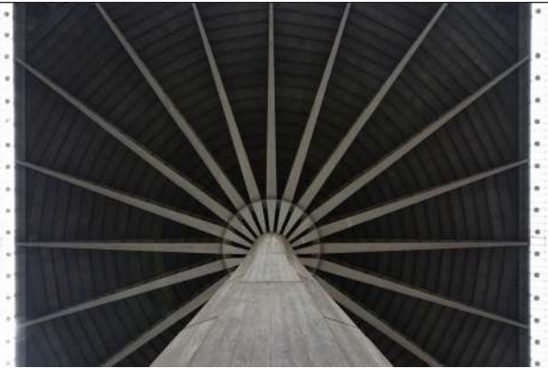
Figure 2.41: Palazzo del Lavoro photo - Main Pillars
