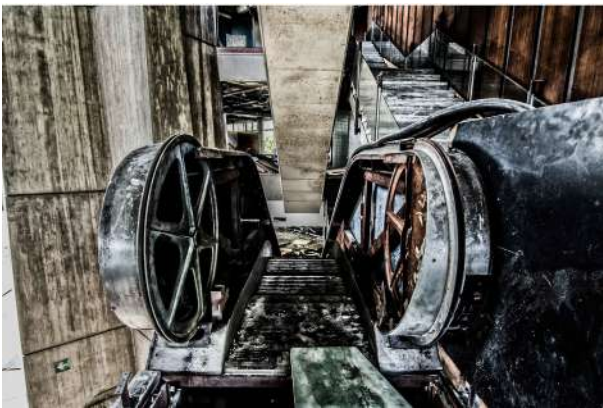
Figure 1.17: Interior after fire devastation.
