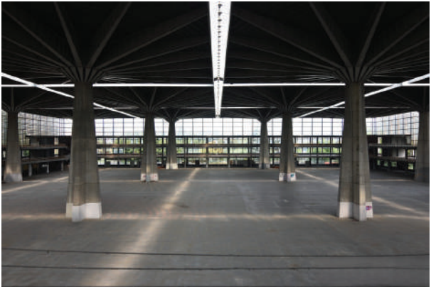
Figure 2.44: Palazzo del Lavoro photo - Interior view from the 2nd level.
