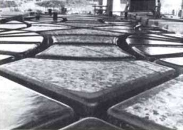
Figure 3.13: Historical construction photographs illustrating the casting process and geometry of the monumental reinforced concrete ribbed gallery slabs.
