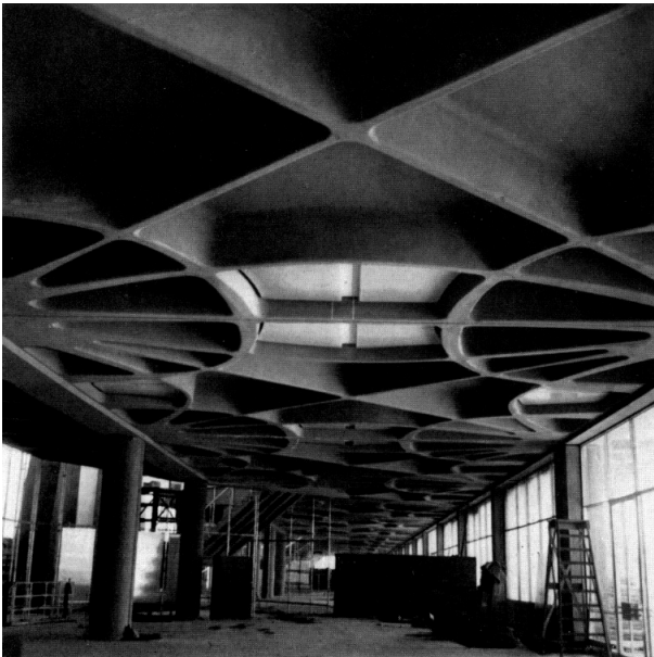
Figure 2.24: Ground floor ceiling
