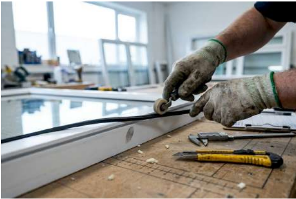
Figure 3.21: Manual installation of high-elasticity EPDM profiles using dry-glazing roller tools to establish a flexible, UV-resistant mechanical buffer zone.
