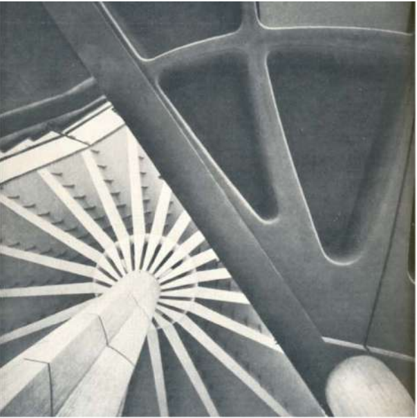
Figure 2.25: Direct photograph showing the ground floor ceiling and the main roof
