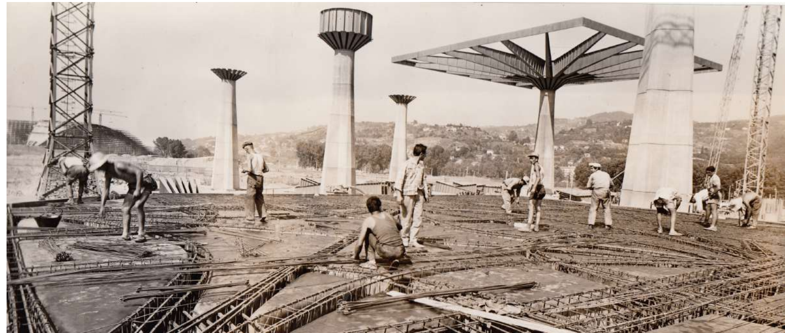
Figure 1.10: Palazzo del lavoro under construction "Courtesy of Fondazione MAIRE - ETS. Materials from the MAIRE Historical Archive."
