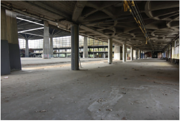
Figure 2.45: Palazzo del Lavoro photo - Ground floor ceiling
