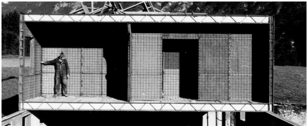
Figure 0.7: Left: "Block-Volume" laid on formwork panels forming the basement floor. Middle: production and assembly of a "Block-Volume" element forming part of the villas plastered in the factory in the post-1985 period. Right: tipping of the "Block-Volume" using an overhead crane.
