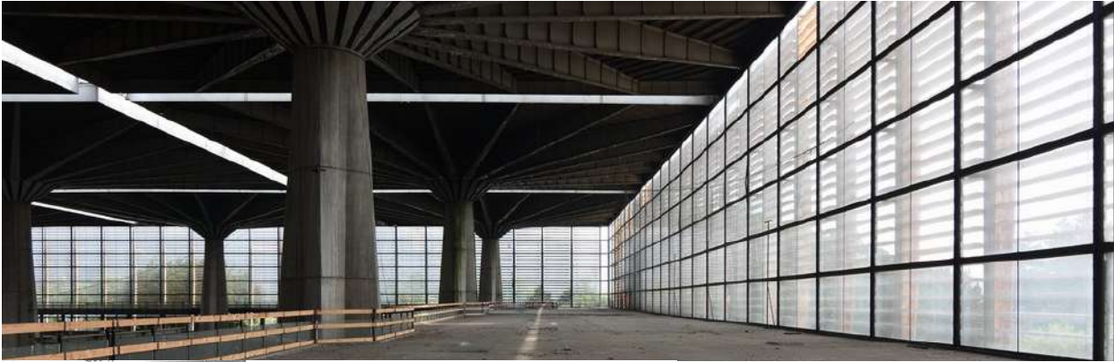
Figure 2.29: Photograph taken on the second perimeter floor visualizing the curtain walls and framings.
