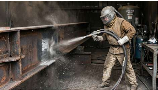
Figure 3.19: Controlled abrasive blasting using aluminum oxide media on structural steel to achieve an Sa 2½ surface preparation grade prior to the application of the high-durability coating system.
