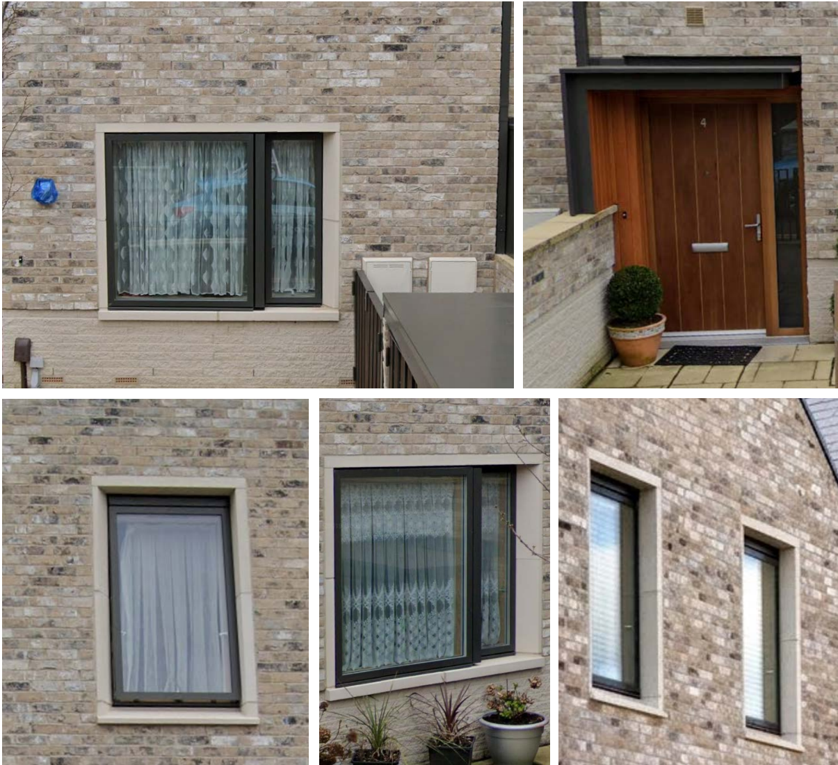
Figure 4.55 Window and door typologies of the case-study building, Darwell Close, Newham, London (Source: Adapted from Google Earth imagery, Google, 2024; edited by the author).
