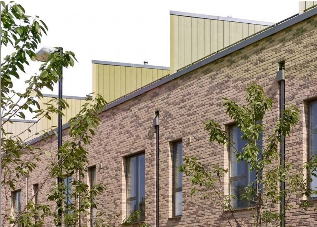
Figure 4.60 Detail view of the Newham Housing case study, illustrating the façade materials, window composition, and roof profile (Source: Bell Phillips Architects).
