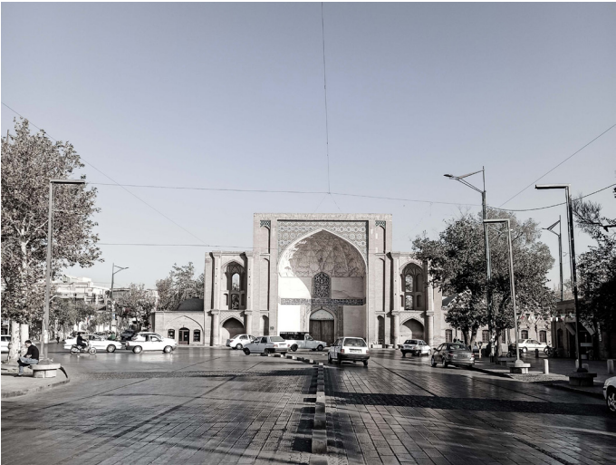
Figure.30 Ali Ghapou Gate, Qazvin, Iran. Main entrance to the garden, view from Sepah street (Khiaban st.)
