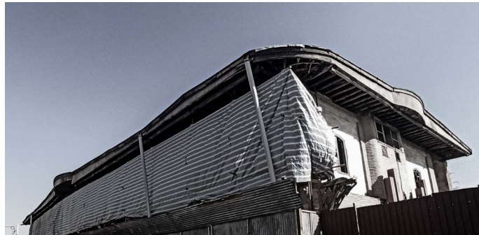
Figure.31 Grand hotel, Qazvin, Iran. View from Peygambaryeh street, Under renovation process to restore the building.
