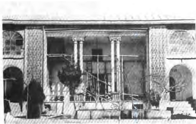
Figure.35 Peghambarieh entrance, south elevation. Befor restoration in Qazar era.
