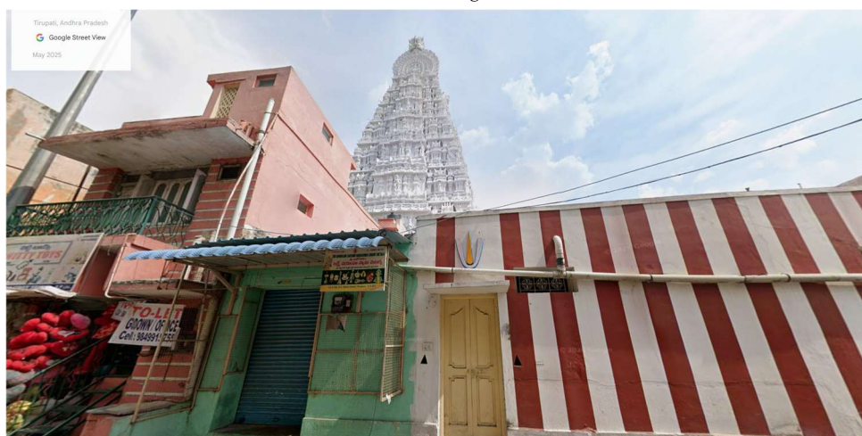
Figure 67: temple, stores, sharing common walls and forming a foreground to the Raja Gopuram Source: Google Street View.
