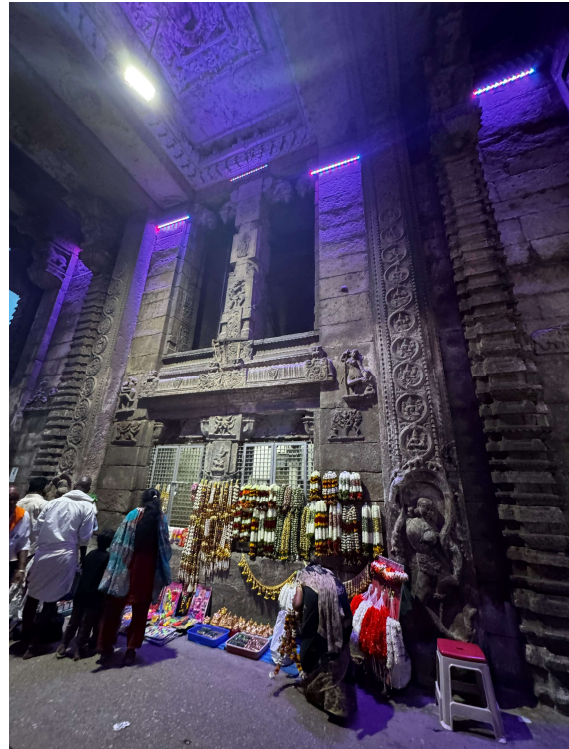
Figure 71: Entrance walls being used by local vendors to hang their items, captured by Author.
