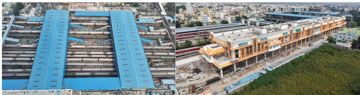
Figure 50: Tirupati Railway Station Redevelopment progress till 30 March 2026. Source: Ministry of Railways, Government of India.
