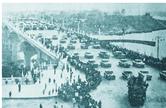
Figure 2-5. On September 28, 1964, the Yongjiang Bridge held its opening ceremony. The bridge is 394.6 meters long and 24 meters wide. Aug 30, 2025. https://www.gxcic.net/article/ab811fb9b4c42ffdce7310ee77c333ac
