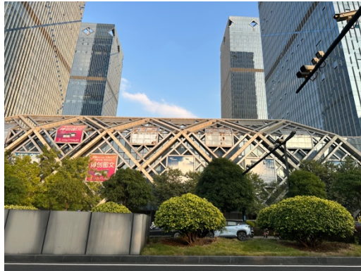
Figure 4-30. Large-scale outdoor advertisement integrated into the architectural structure along a primary arterial road in Wuxiang New District, designed for long-distance visibility and city-image presentation.
