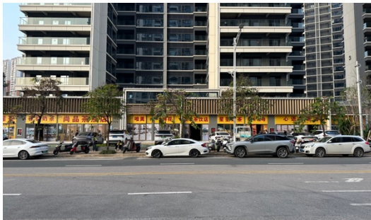
Figure 4-25. Ground-floor frontage dominated by enclosed commercial forms in Wuxiang New District, contrasting with fine-grained and permeable street edges in urban villages and historic districts.
