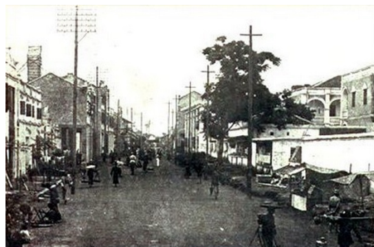
Figure 2-3. Reconstruction of Nanning Zhongshan Road
