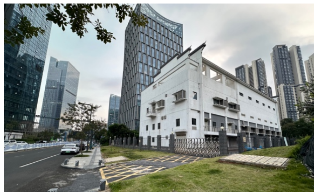
Figure 4-21. A substation integrated into the streetscape through planning control and image-oriented design.
