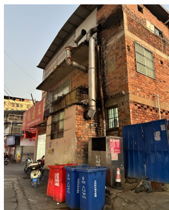
Figure 4-6. Illegal restaurant extensions and exposed waste-management infrastructure.
