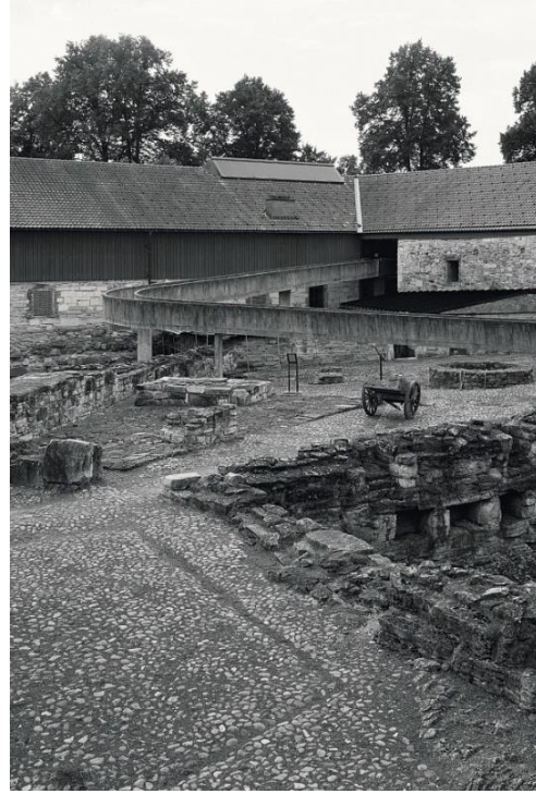
Figure 5-8 Ramp Traversing the Site and Barn
