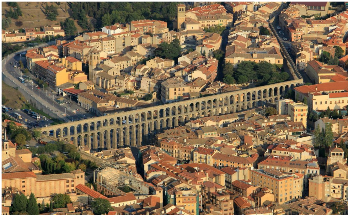
Figure 1-1 Aerial View of Segovia.
