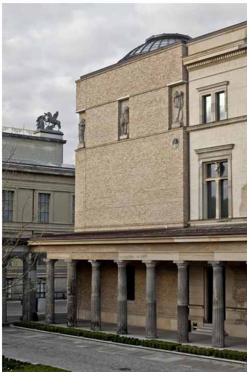
Figure 5-5 Juxtaposition of the Building Façade and Materials
