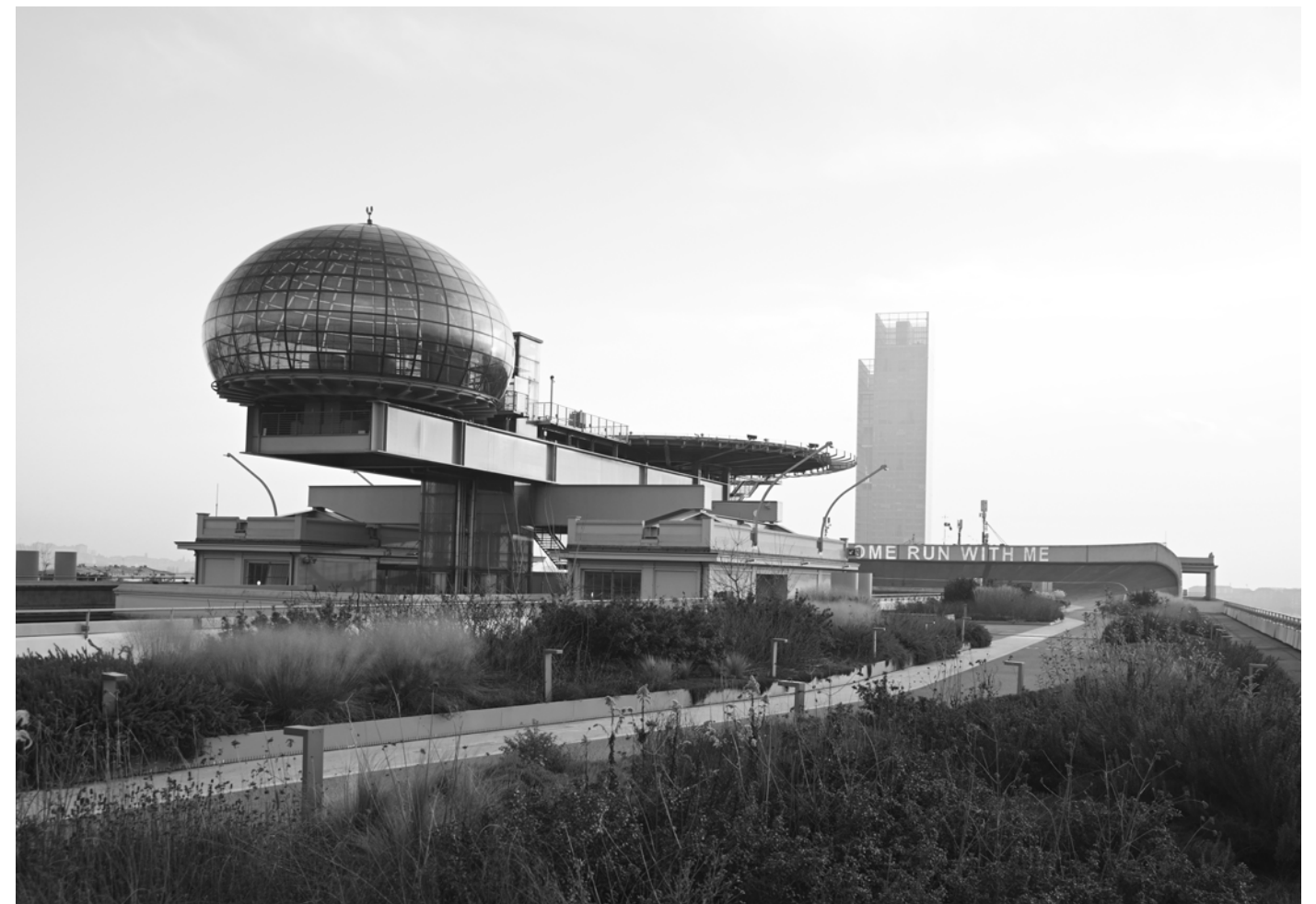
Image 30 : Roof of Lingotto
