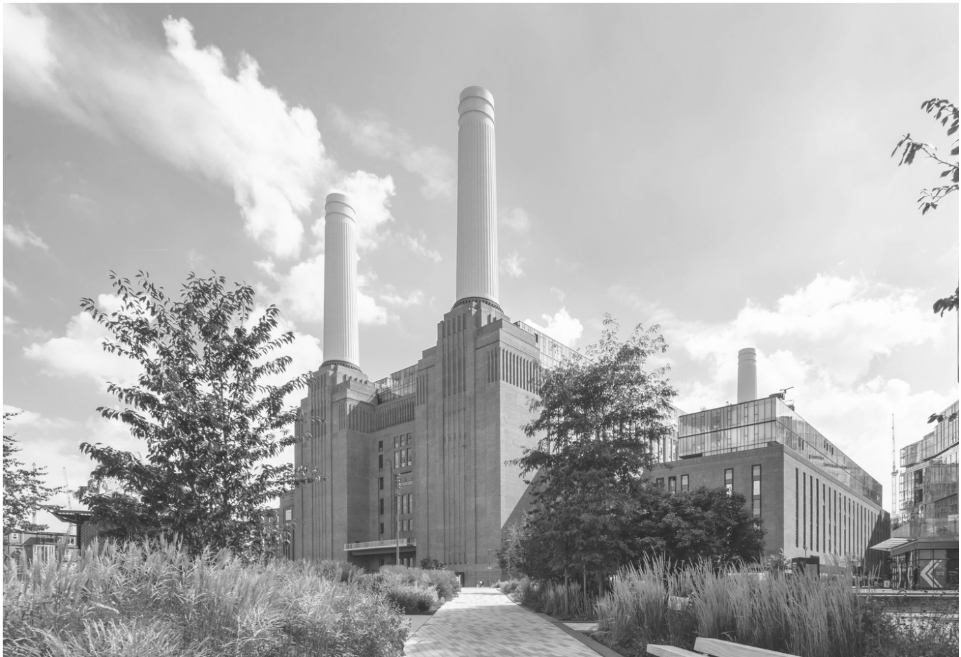
Image 8 : Battersea Power Station /Paula Pintos
