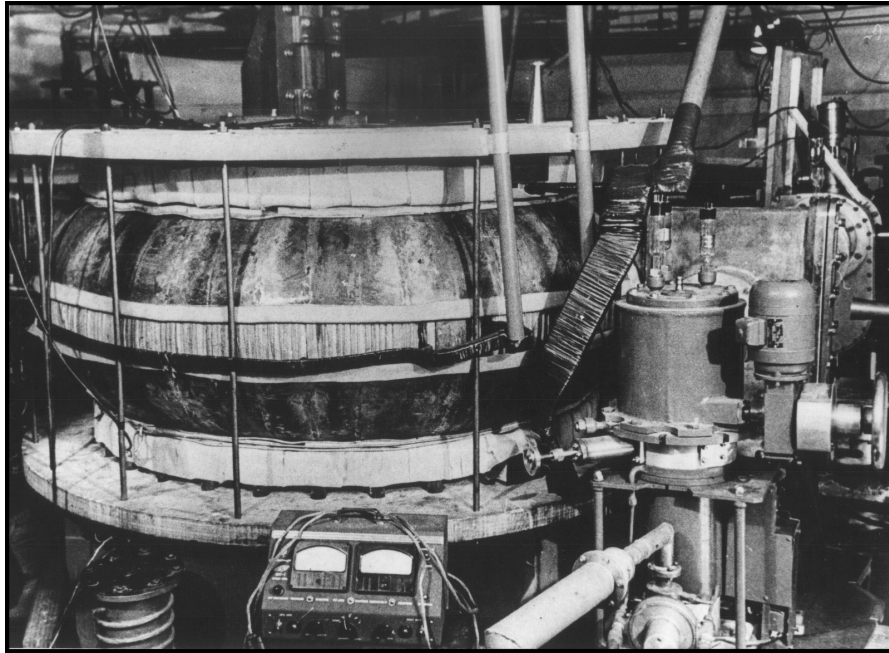
Figure 1.8: World's first tokamak device: Russian T1 tokamak
