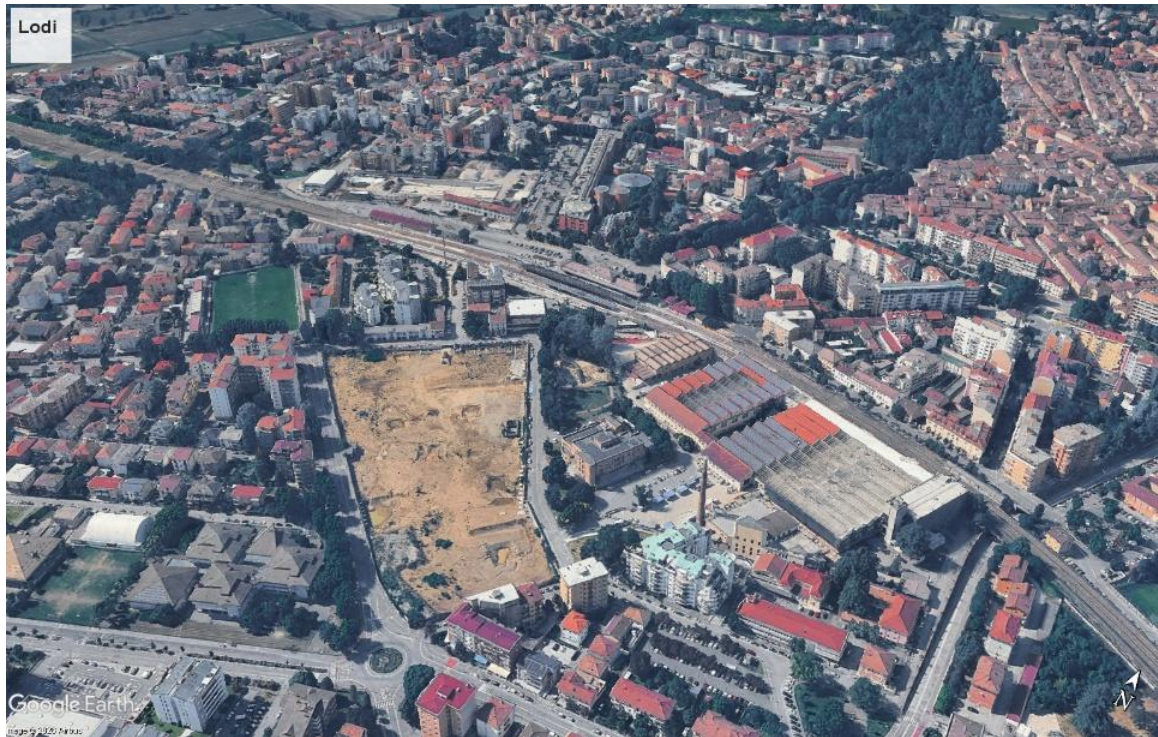
Figure 15 – Satellite view of the Lodi station area showing dominant residential areas with substantial non-residential lots within the catchment areas. Map data ©2025 Google.
