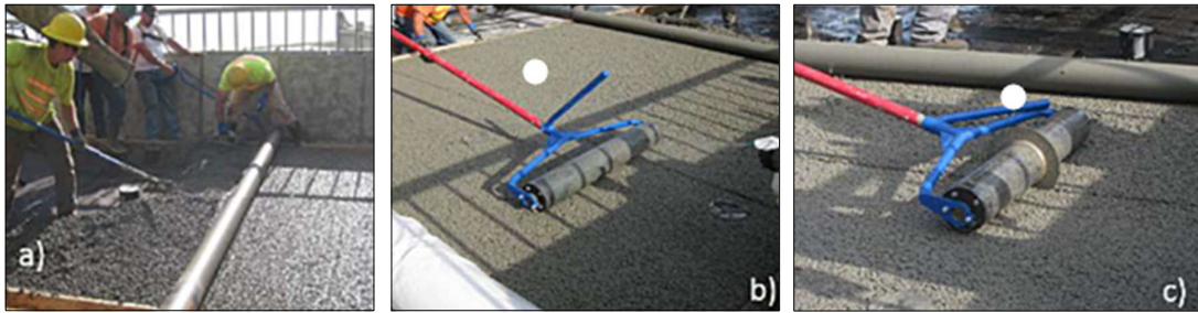
Figure 1.2: Field demonstration of the porous concrete placement workflow (adapted from Nassiri et al., 2017)
