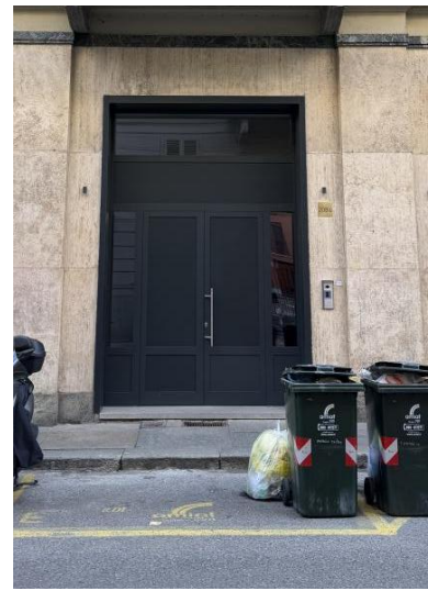
External solid metal door at No. 20, Via Principe Amedeo, newly added.
